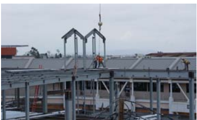
Science Building Topping Out
